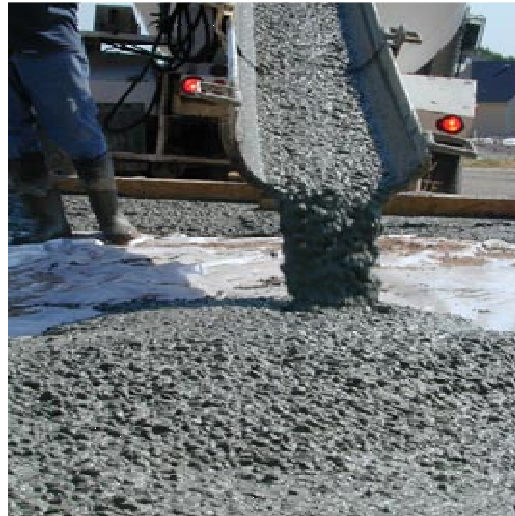
Placement of Colored Concrete
